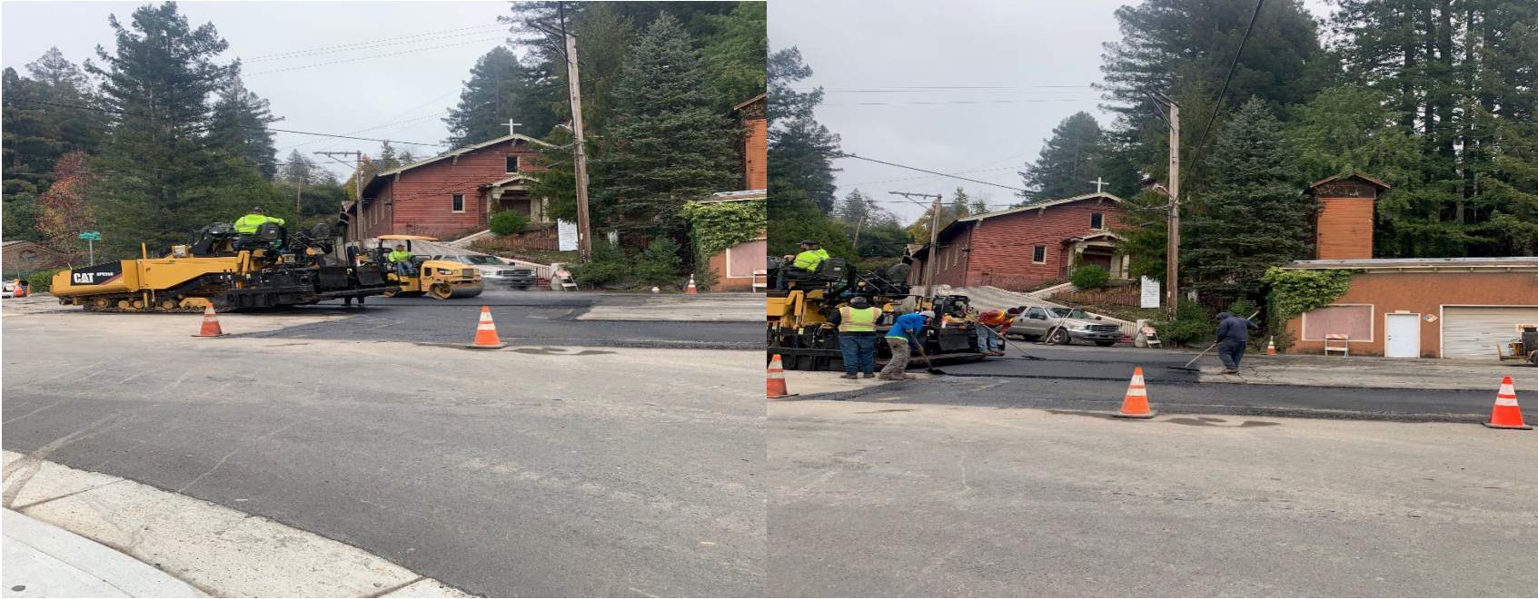
Paving Armstrong Woods Road
